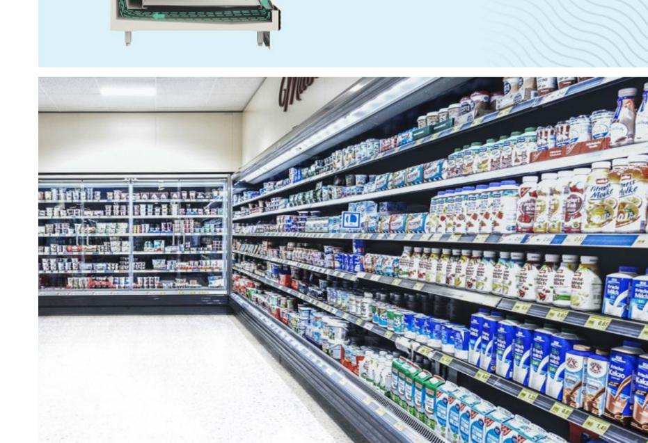
The cool airflow is separated into two air curtains inner and outer air curtains.
